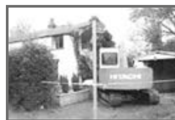
SNOWDROP COTTAGE BEING DEMOLISHED FEB 2008
